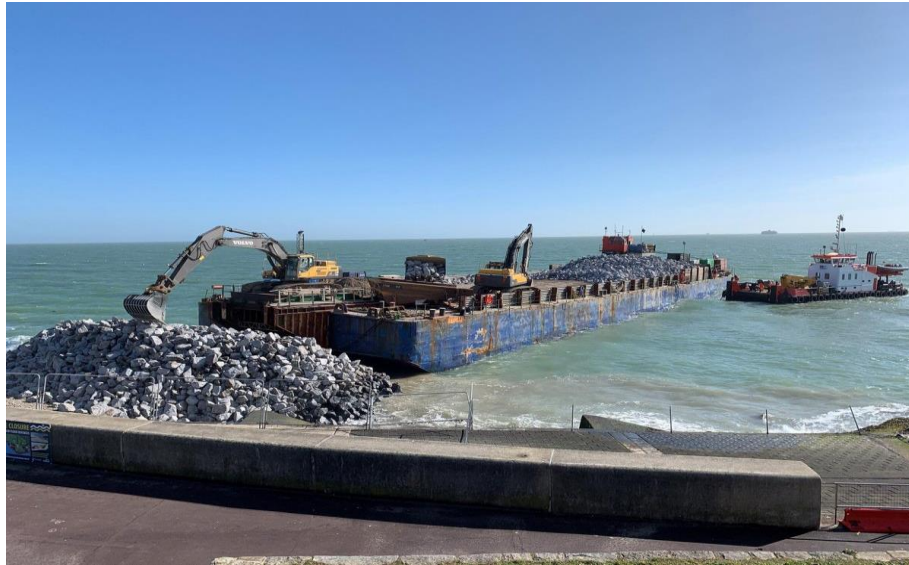
Delivery of rock armour to Southsea
