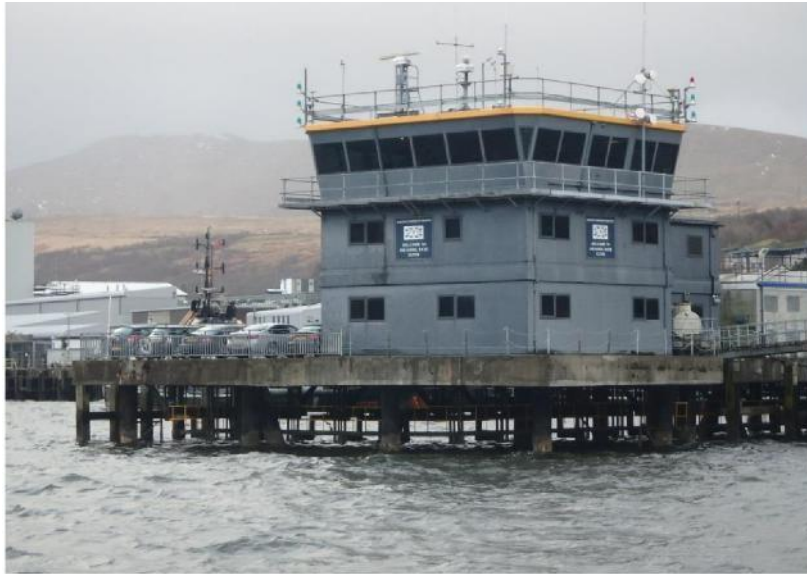
Figure 2 – KHM Renown Building, HMNB Clyde
